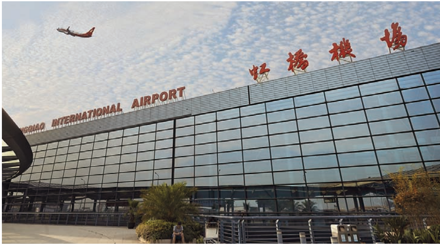
Hongqiao International Airport in Shanghai. — CFP
